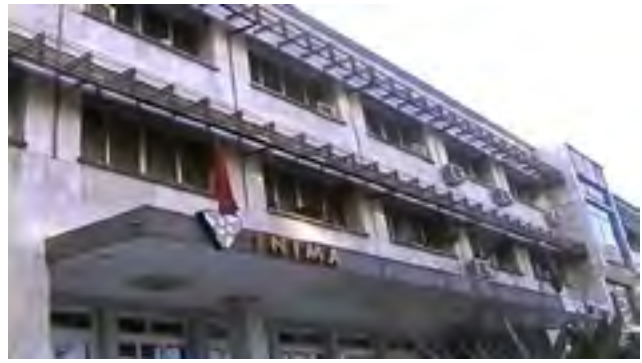
Fig. 3 – Front view of INIMA building
